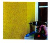
Screw the object to be mounted in the MTH ELEMENTO DI FISSAGGIO INTERNO SPALLETTA Tra-Wik-PH internal jamb. The screw depth into the bracket must be at least 26 mm. This ensures that the entire thickness of the phenolic resin plate is fastened correctly.
