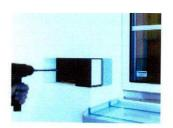
Cover the heads of the fixing screws with insulating material covered with adhesive mortar and press until flush with the rest of the insulating material.
